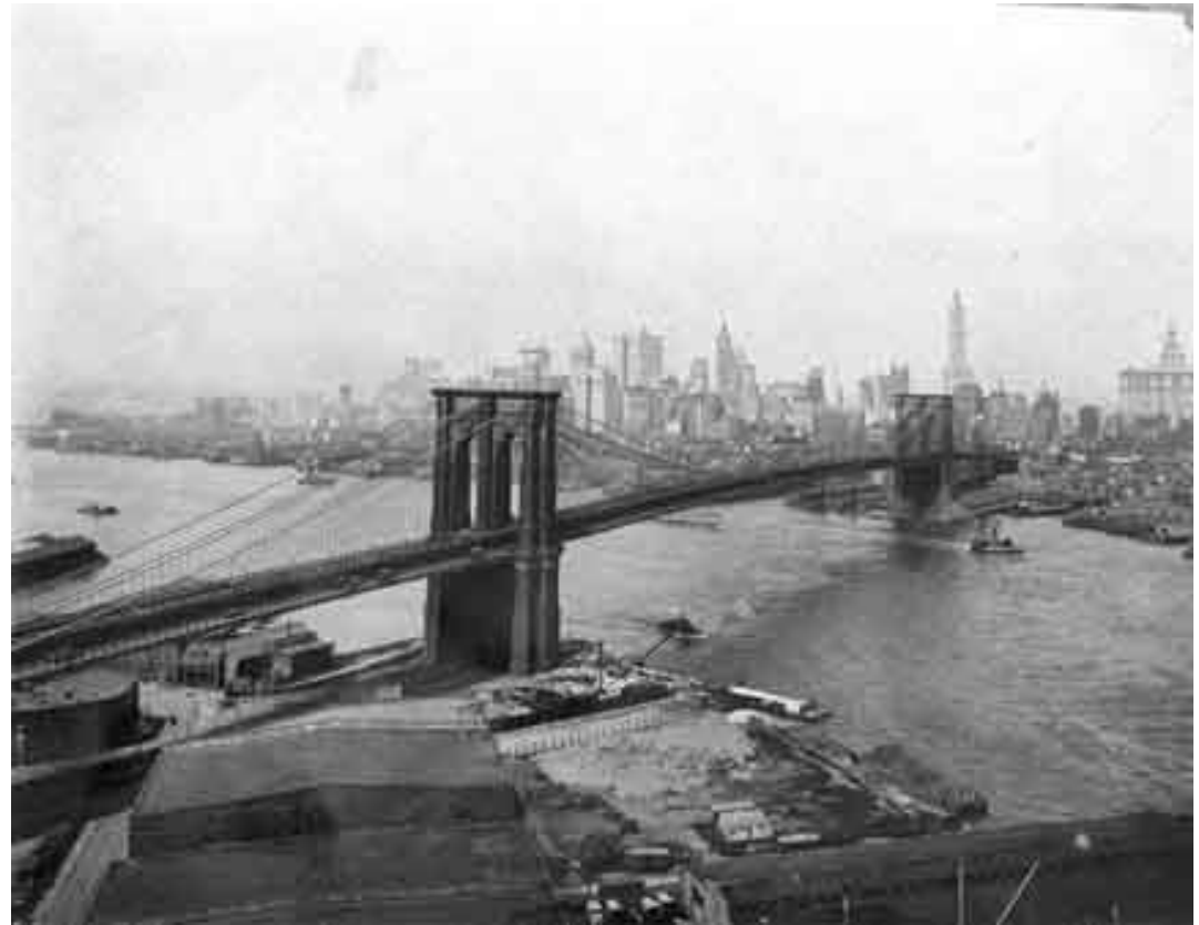
Brooklyn Bridge, New York City
