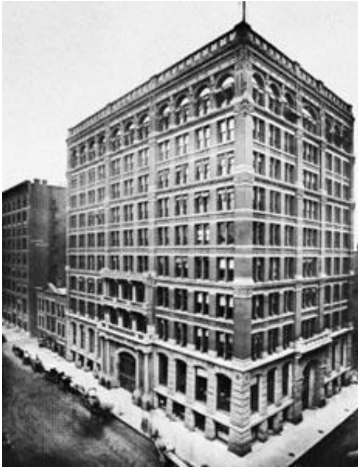
Home Insurance Building, Chicago
